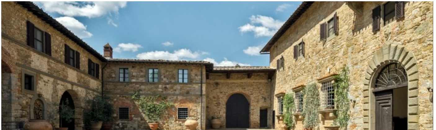
THE INNER COURTYARD — STONE, LIGHT, CONTINUITY
